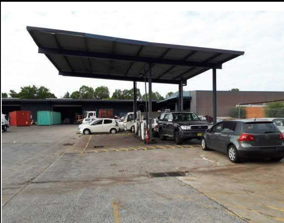
Photograph 7 – View of unused refuelling station
