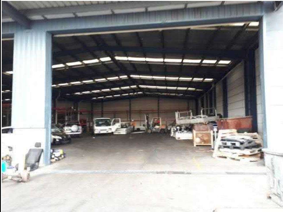
Photograph 16 – View of warehouse in the southwestern portion of the site
