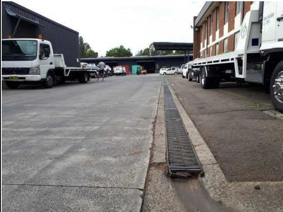
Photograph 4 – View of northern portion of the site near the main office
