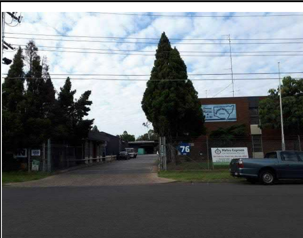
Photograph 1 –View of front entrance from Seville Street
